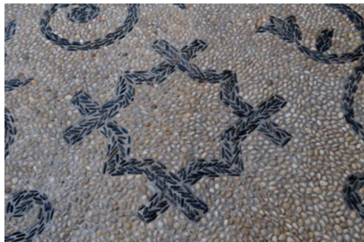
1, 2. Various decorative patterns of traditional Granada cobbled pavements 3. Traditional cobbled pavement in Placeta del Comino, Granada
