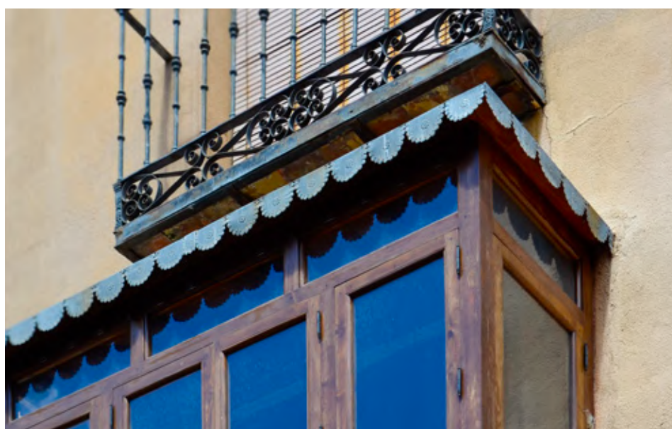
Metal drip moulding above a glazed gallery
