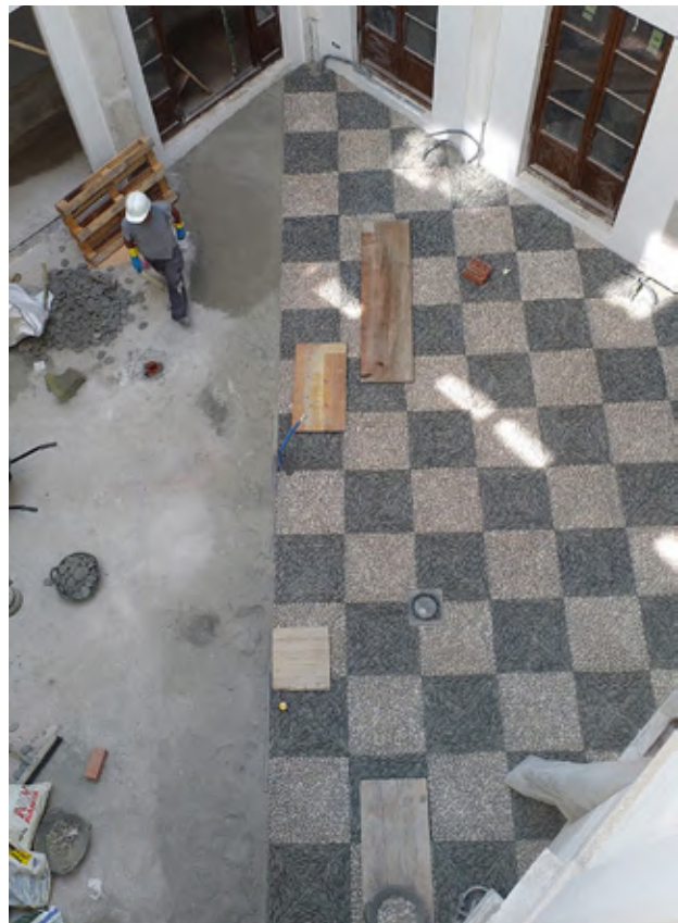
Execution of a traditional cobbled pavement in a Granada courtyard
