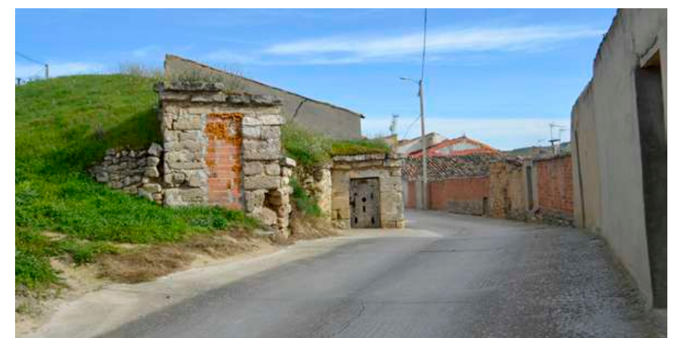
Diverse views of the building and the lot of the intervention site
