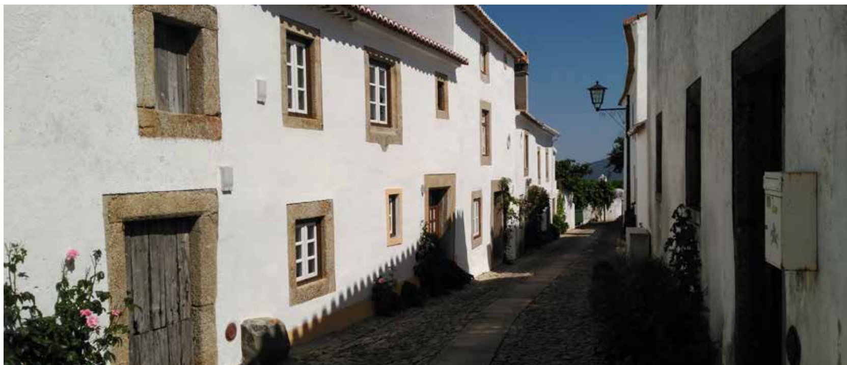
Traditional houses in Marvão
