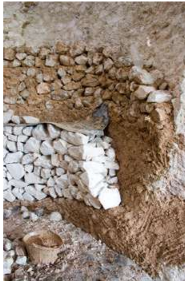
2. Repair of the inside of a traditional lime kiln
