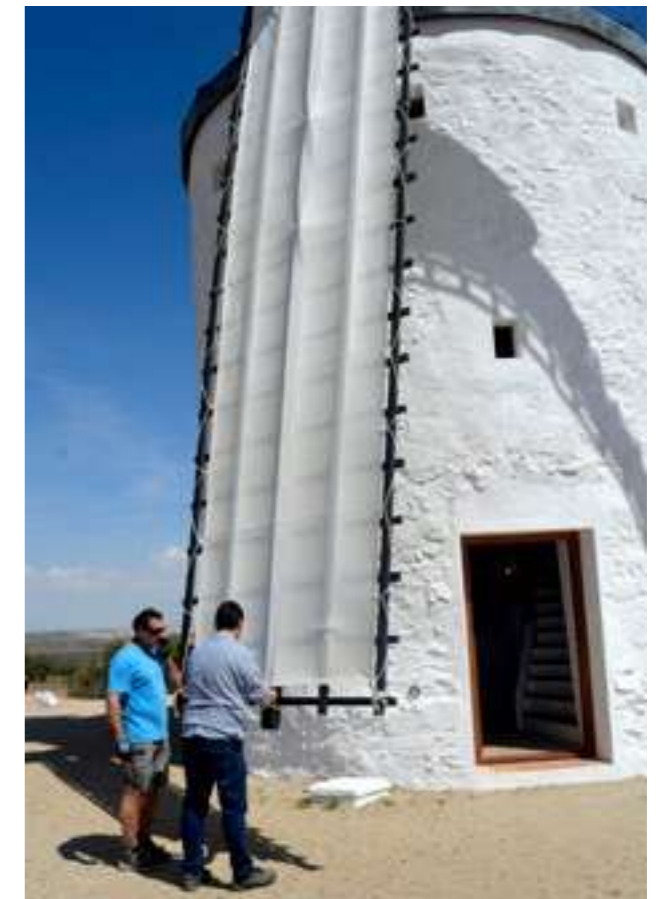
Fitting of sailcloth on the parts of the sails that receive the wind
