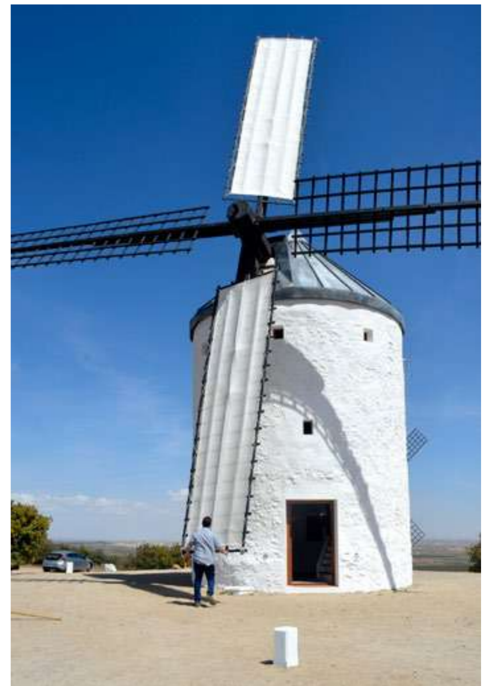
Fitting of sailcloth on the sails of the mill in Puerto Lápice
