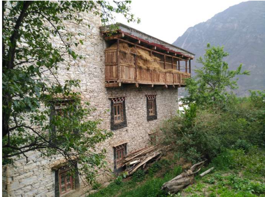
Arquitectura tradicional en Chonglu, Sichuan, China Arquitectura tradicional em Chonglu, Sichuan, China Traditional architecture in Chonglu, Sichuan, China
